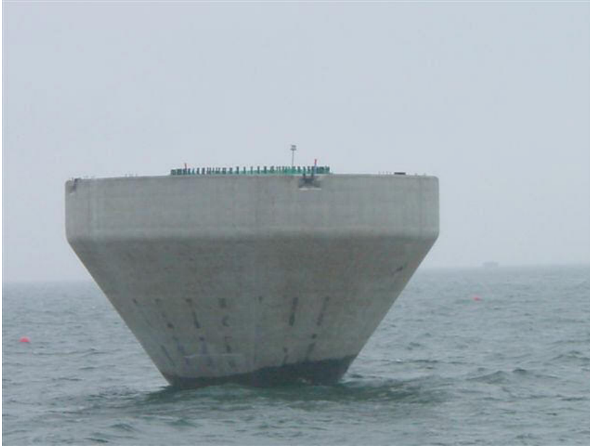
Figure 4. Picture of one of the turbine foundations put in position in the wind farm area.
